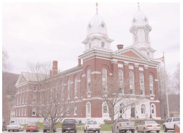
This courthouse roof was unnecessarily condemned and scheduled for replacement. The Vermont "sea green" slate roof is only 72 years old — about halfway through its life. Comprehensive restoration work on this roof will only cost about 10% of the cost for total replacement because the slates and fasteners are still in good condition. Most of the flashings, however, need to be replaced.
