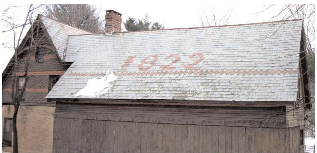
A recent photo of a barn in Vermont testifies to the potential longevity of a standard slate roof.
