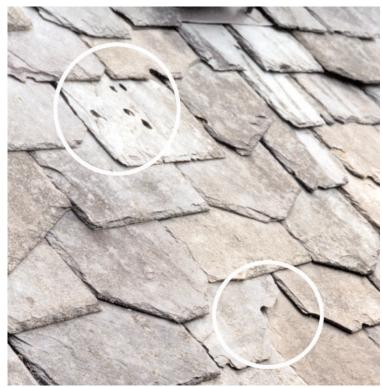
Hail damage of this nature as seen on Chicago area "ragged butt" slate roof is repairable by simply removing the damaged slates and replacing them. Most of the slates are undamaged.
